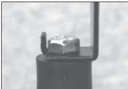
22. Bend the tab on the bracket up. This will keep the Hex bolt from backing out.
