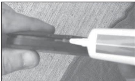
15. Apply sealing grease into the groove of the small plug.
