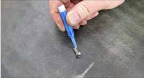
10. Apply one drop of the provided thread locker to the provided filter back plate mounting bolts.
